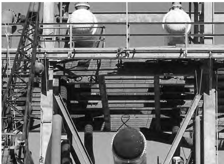
Monokote Z-156PC fireproofing has been designed as a cost-effective fireproofing solution for pipe racks, vessel skirts and other structural supports.
