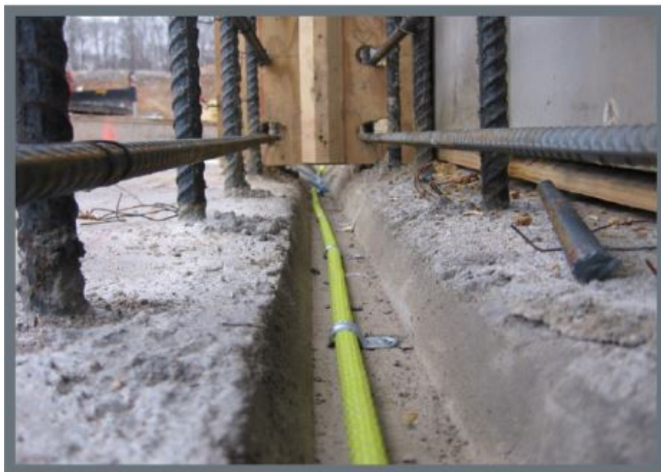
Figure 4. Anchoring clips on INJECTO ®
