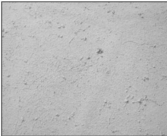
Photo 2. Example of over-mixing.
