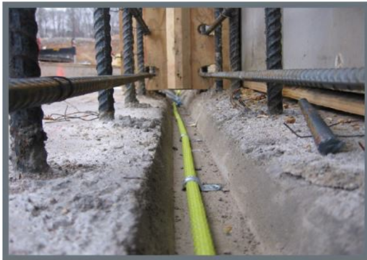
Figure 4. Anchoring clips on INJECTO®
