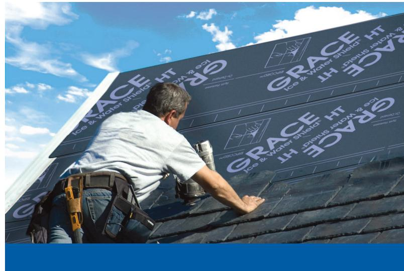
**Ripcord** — Split Release on demand feature makes Grace Ice & Water Shield® HT underlayment easier to apply. Faster application of the membrane in the straight-aways, as well as ease of membrane positioning in detail areas (valleys, around dormers, etc.).
