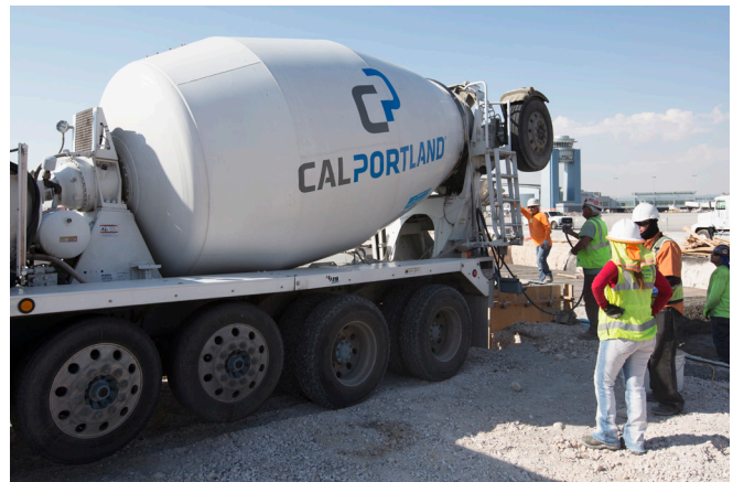
ADVA® water reducing and Eclipse® shrinkage reducing concrete admixtures ensure that the tunnel meets rigorous design criteria.
