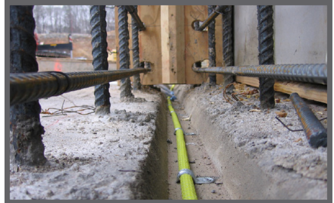
Figure 5. Anchoring clips on Injecto
