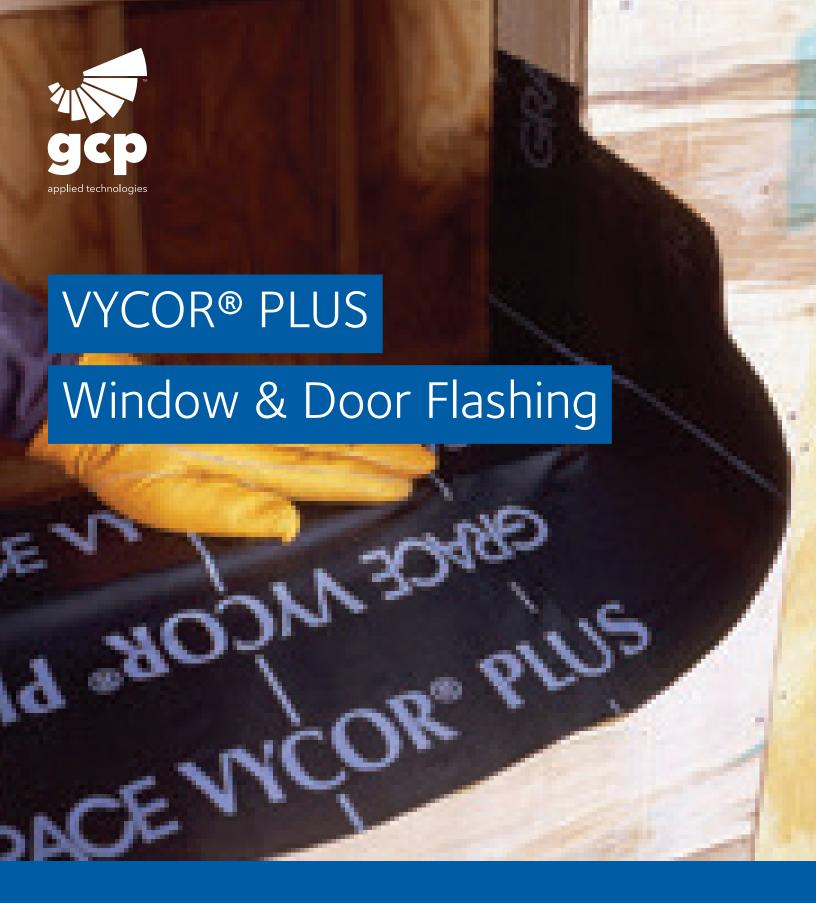
Vycor® Plus is a high performance self-adhered flashing, that provides premium protection against water infiltration in critical details such as windows and doors. When properly installed, Vycor® Plus flashing reduces the risk of mold and rot development, and contributes to energy efficiency.
