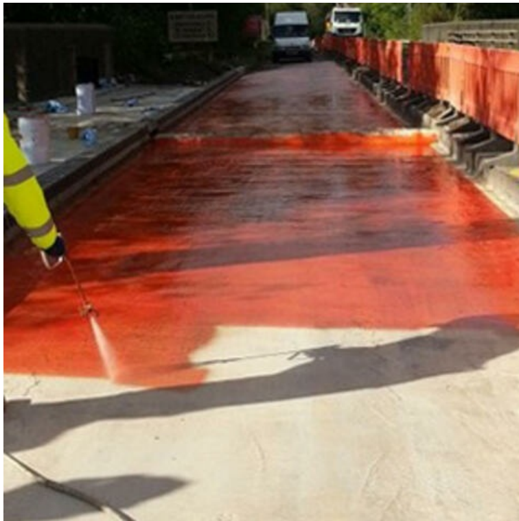
Crumlin Bridge Protected with Spray Applied Waterproofing
